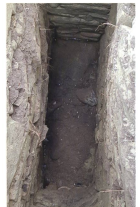
23 Bolligen, Manneberg, Reservoir
