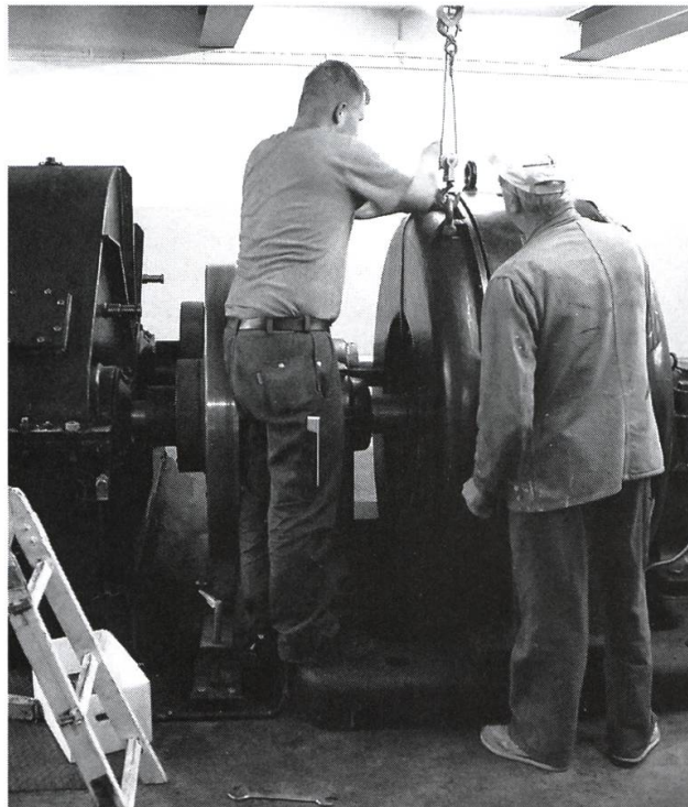
Renovation des Generators.
