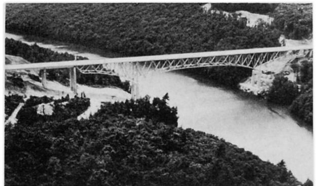
13. Clarion River Bridge on I-80
