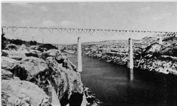
10. Pecos River Bridge
