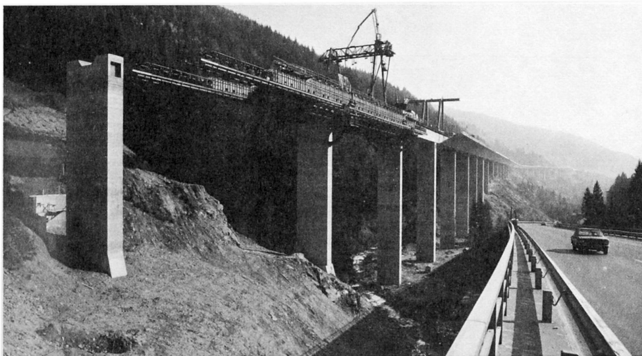
L 22 with launching girder
