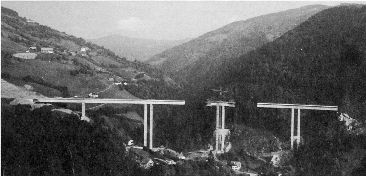
L 23 under construction
