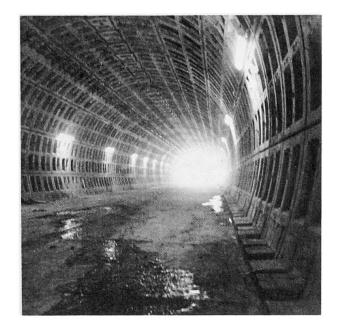
Tunnel driving commenced in January 1979. During the first year of driving an average production of 18 rings per week was achieved representing 21.6 m complete with road deck. During a period from August 1979 until the end of February 1980, an average advance of 30 m per week was maintained.
