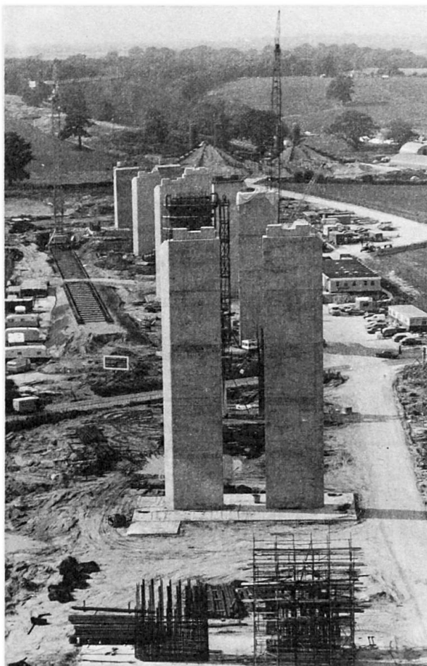
Viaduct piers – August 1980
