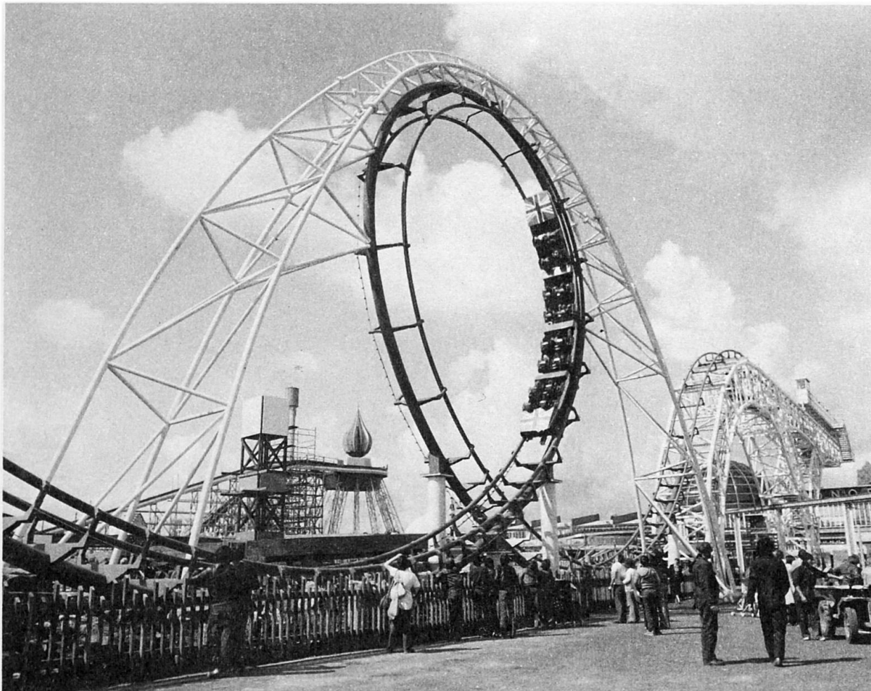
Fig. 2 Central loop and arch
