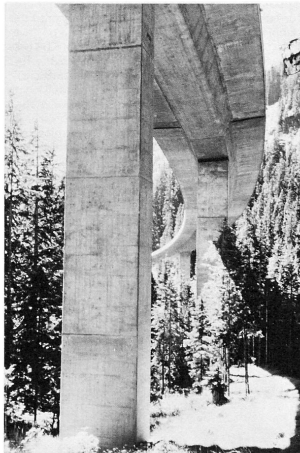
Fig. 5 Denny Creek Bridge
