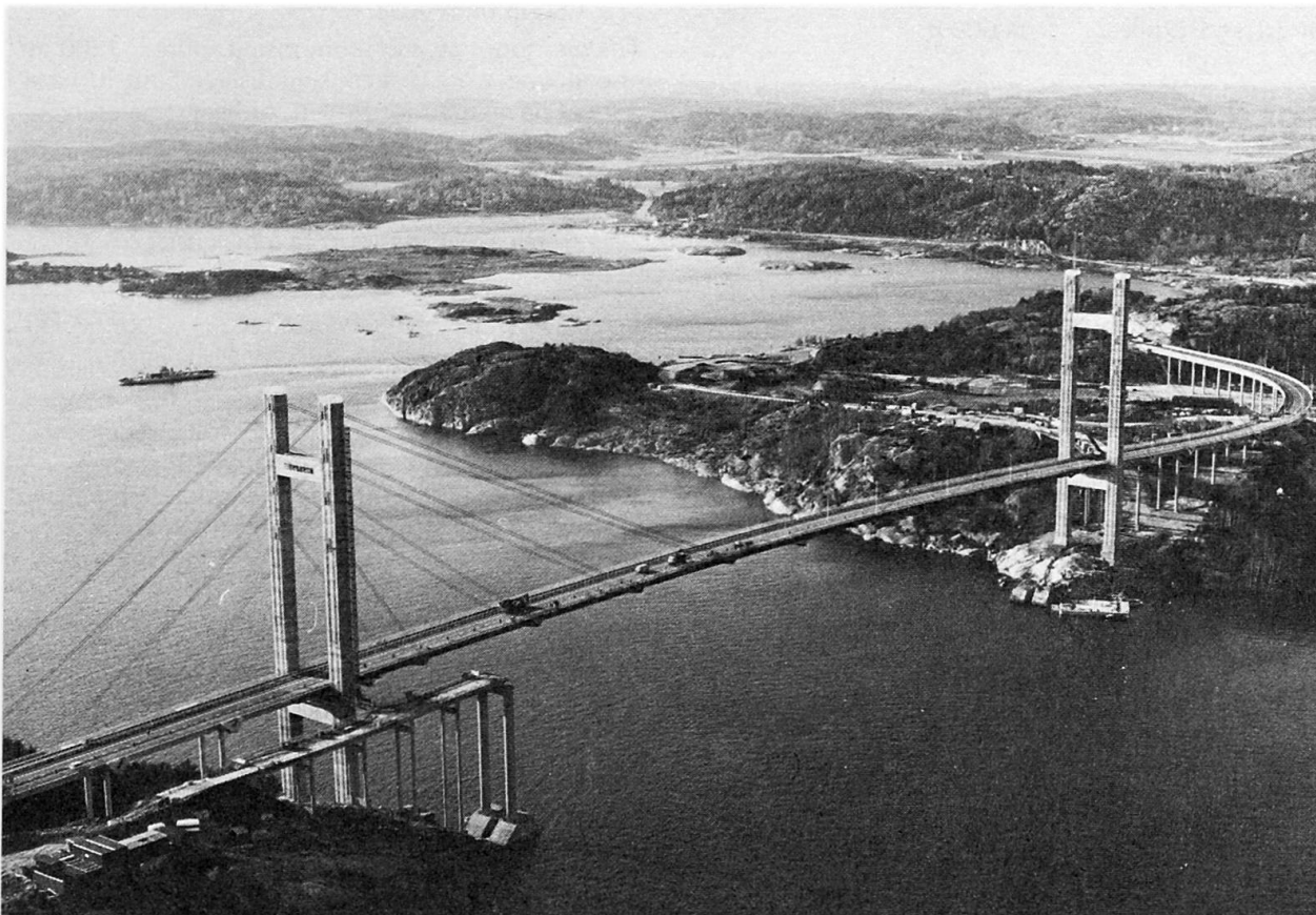
Fig. 3. The finished bridge
