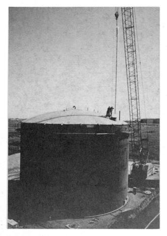
ted 100 % standard proctor. Laying of floor plates started in December, 1982. The plates were lapped and welded sloping toward a small central steel sump. Tank wall construction started in the new year.
