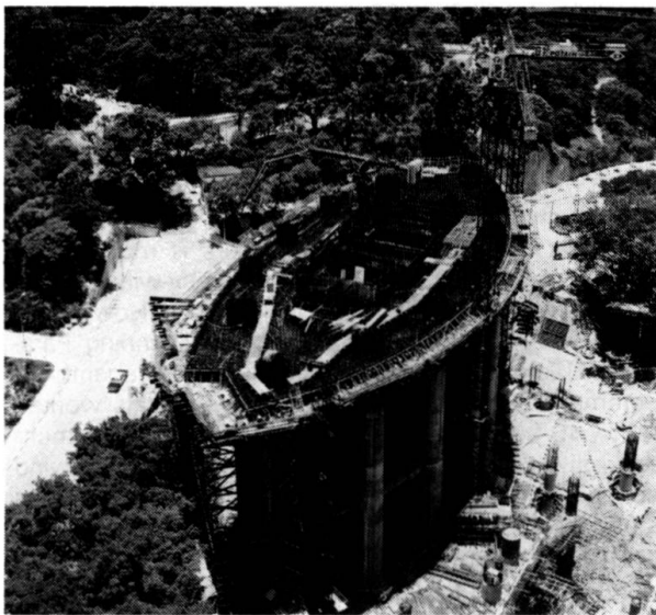
Fig. 4 Transfer plate of Tower B under construction (June 1988)
