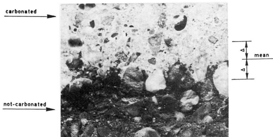
Fig. 7 Irregular carbonation front in concrete
