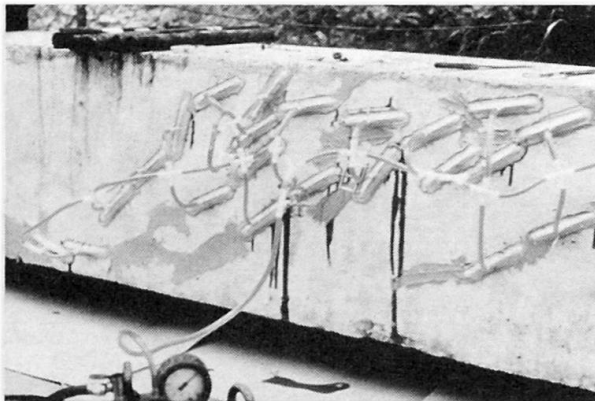
Fig. 18 Example of Crack Grouting
