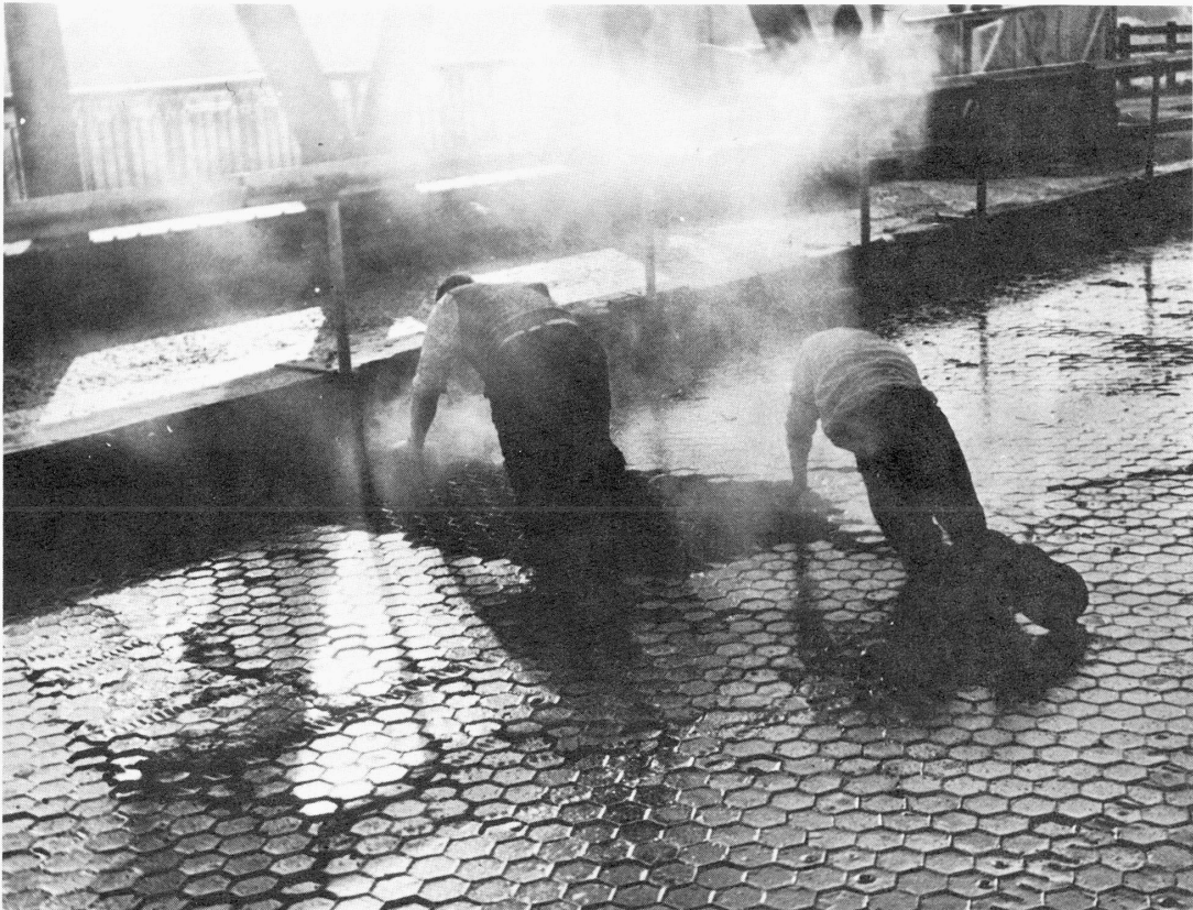
FIG. 1 HEXAGONAL GRID 1 in (25 mm) DEEP, ON AN ALUMINIUM DECK OF A BASCULE BRIDGE IN HULL.
