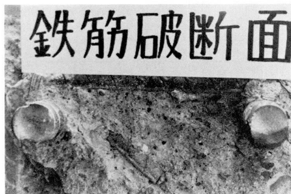
Photo. 2 Fracture Surface of Bar
