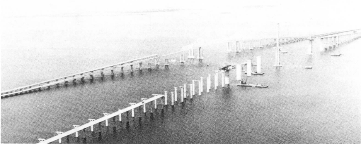
Fig. 1.1 Construction of the new Sunshine Skyway Bridge.
