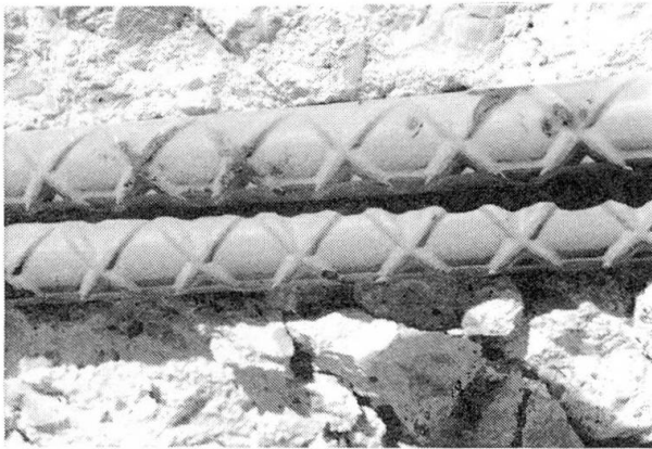
(b) Epoxy-coated bars
