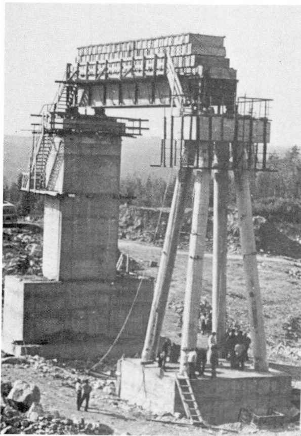
Fig.1. General view of the railway bridge section model
