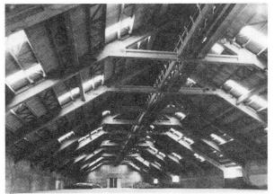
precast concrete elements proved to be much more economical and durable for the corrosive atmosphere inside fertiliser storage structures.
