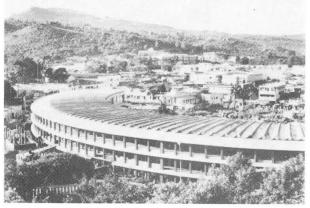
The pre-stressed channels are supported on brackets projecting from the RCC core walls, in a step-like fashion and form the upper gallery. The gallery steps are finished with marble. The lower gallery is formed by filling with earth and topping with PCC. Cut-outs in the core walls serve as passage for connecting the different compartments. (Fig. 7)
