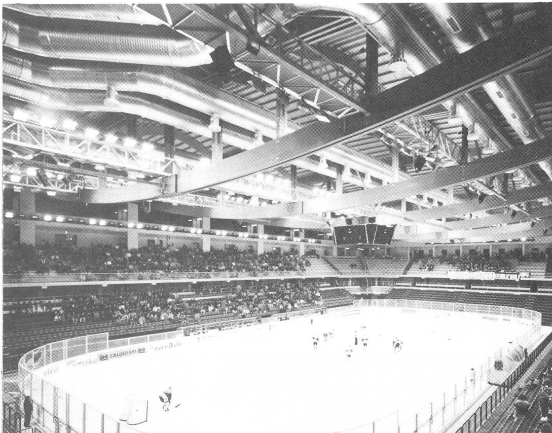
Fig.3 "Wave" Stadium. The new ice hockey arena in Bolzano.
