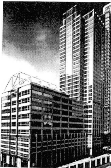
Fig. 6. Morton International Building
