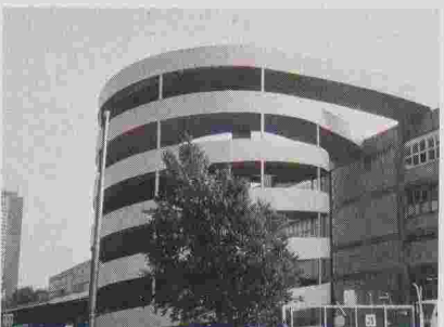
Rampe de parking Migros Herdern
