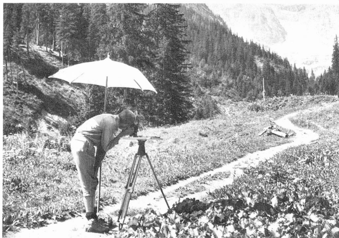
Topographical details were surveyed using the planetable
