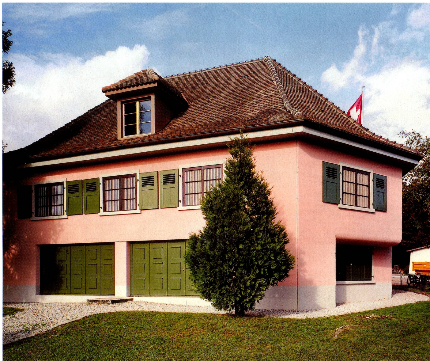
Villa, 1940, infantry bunker, Gland VD: solid construction with tiled hip roof and dormer window. Behind the template windows, curtains are painted directly onto concrete. The bunker is now used as a museum.
