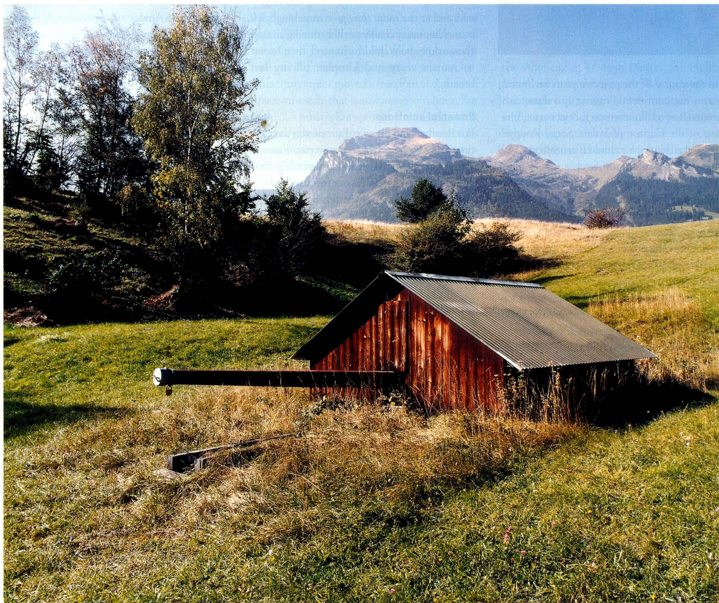
Hut, 1939–43, armoured turret of the Magletsch fortress, Oberschan SG: The turret is covered with planking and a corrugated metal roof. The tank gun barrel is not camouflaged and the mouth is covered.
