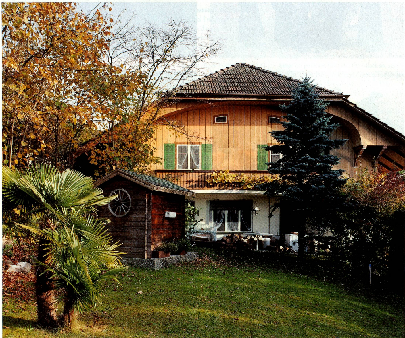
Chalet, 1941, infantry bunker, Hilterfingen BE: concrete building with tiled saddle roof and overhang. Windows, shutters and balcony balustrade are painted on wood cladding. Under the balcony is the bunker entrance, disguised as a window with the roller blinds half-closed.
