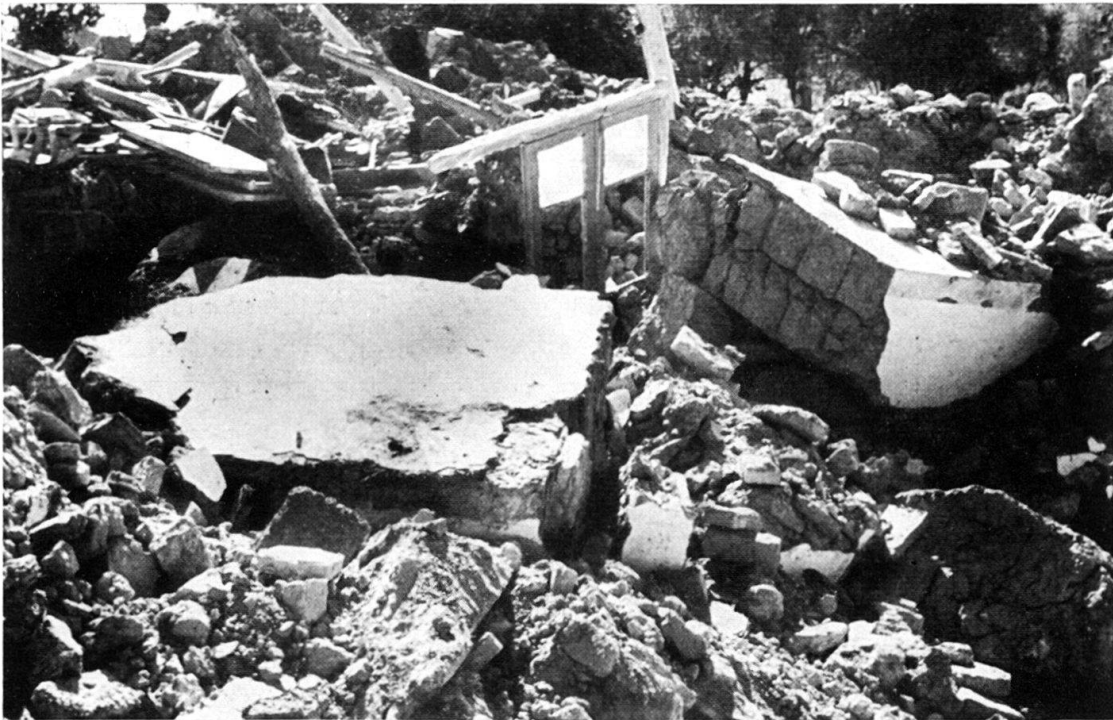
Fig. 17. Total destruction in Kakhk.
