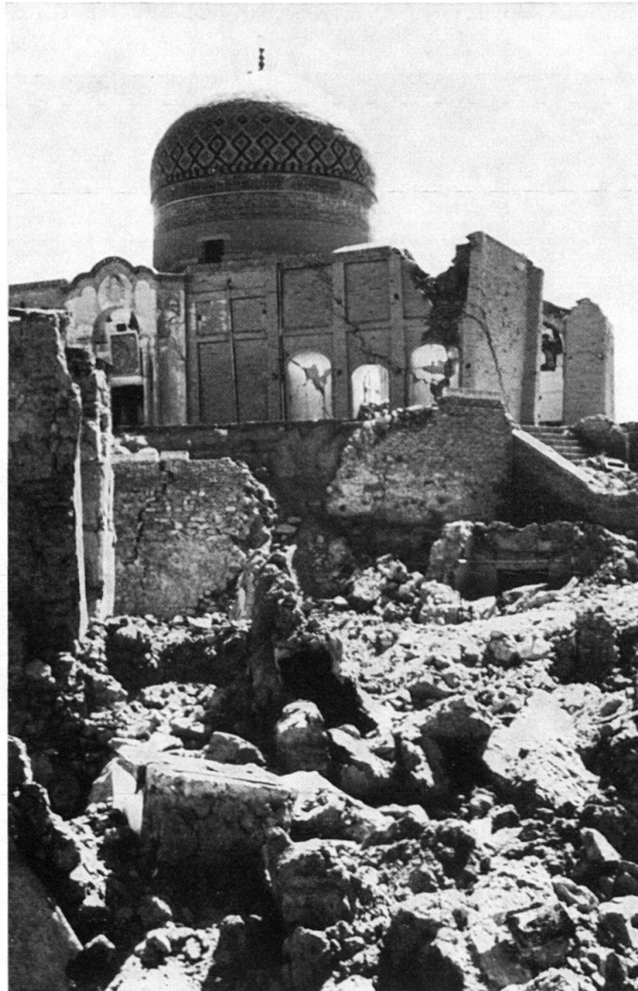
Fig. 18. The undamaged cupola of Kakhk mosque.
