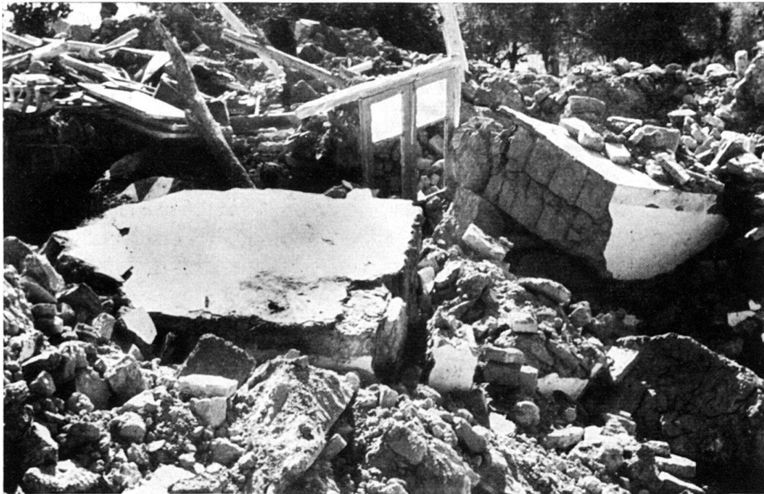
Fig. 17. Total destruction in Kakhk.
