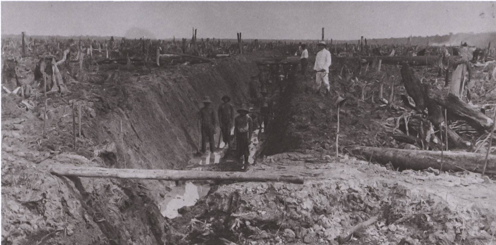
4 Clearing of tropical forest on the plantation Telok Pandjie in Sumatra, 1918.
