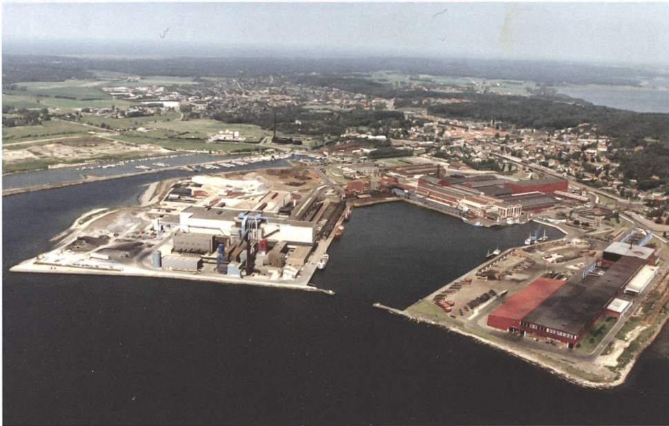
3 The Danish Steel Rolling Mill, Frederiksværk. The oldest part of the steelworks is in the middle. Built on the landfill from the furnaces is a rolling mill for long products (right), and the 1975 electric arc furnace from 1975 (left).
