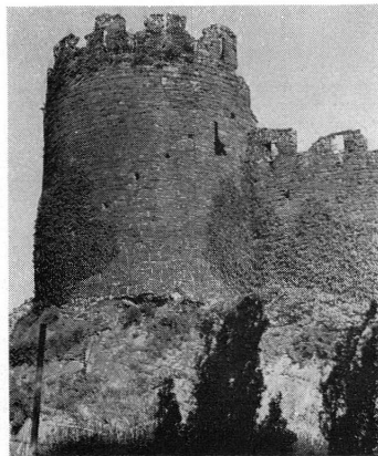
Plate I. Helicoidal scaffolding . - 1. Conway Town Walls, Tower No. 15 (1283-4). - 2. Harlech Castle, S. W. Tower (c. 1289). - 3. Saxon (Valais), Donjon (1279-80). - 4. Conway Castle, Prison Tower (1283-6). - 5. Saillon (Valais), Donjon (1261-62). - 6. Conway Town Walls, Mill Gate, Round Tower of King's Wardrobe (1285-6). - 7. Conway Town Walls, Watch Tower (1283-4). - 8. Conway Town Walls, Upper Gate (1283-4).
