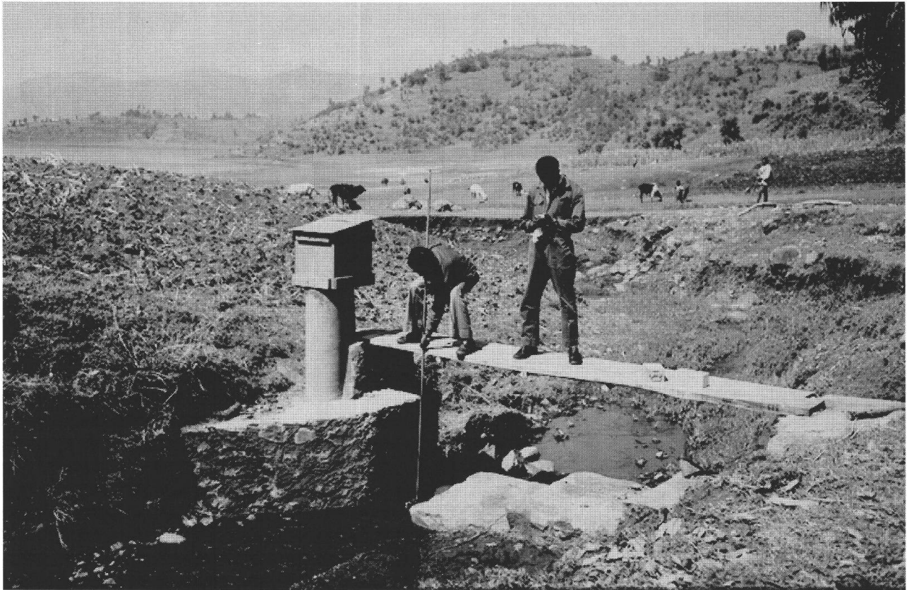
Fig. 2: Long-term monitoring of natural resource processes to gain a better understanding of the dynamics of global and local change. Catchment runoff and sediment loss are being assessed by the Institute in Maybar, Ethiopia.
