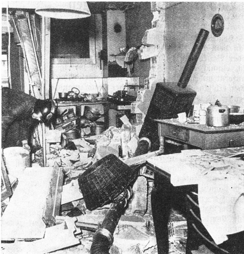
Gasexplosion in Bern
