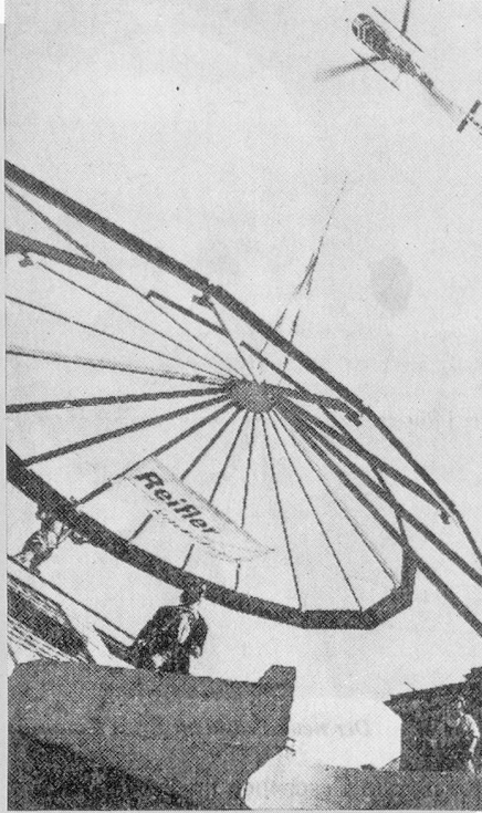
In a spectacular move, a glass dome was placed by helicopter on the top of the building housing Orell Füssli's mammoth book store.
