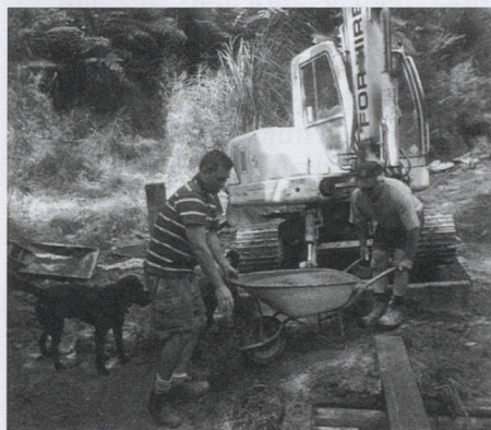
Bridge repairs Swiss farm
