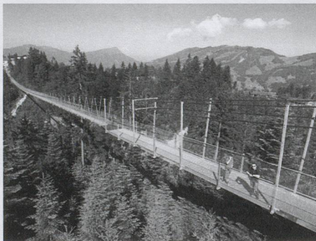
Skywalk suspension bridge
