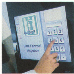
1-3 The European Norm EN81-70 describes how a lift for people with disabilities must be constructed.
