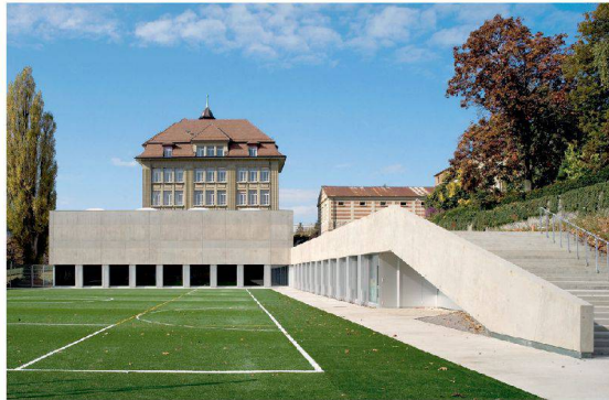
43 Sporthalle Gymnasium Beaulieu
