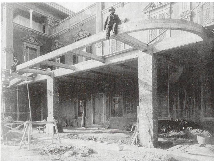
Quarto, Villa Quartara, 1905–06, Auskragung in Eisenbeton System Hennebique. (Repro, S.172)
