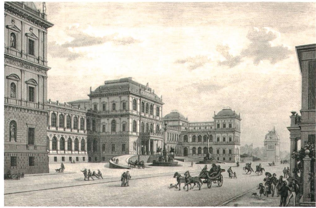
Fig. 4 The new art academy building in Munich, 1883, reproduction (P. Meurer, X. A., Berlin) after a drawing by the architect Gottfried von Neureuther, in Deutsche Bauzeitung 17(6), 1883. Photographic paper mounted on board, 16.3 × 23.9 cm, Architectural Museum of the Technical University, Munich, inv. no. neur_g-213-51.
