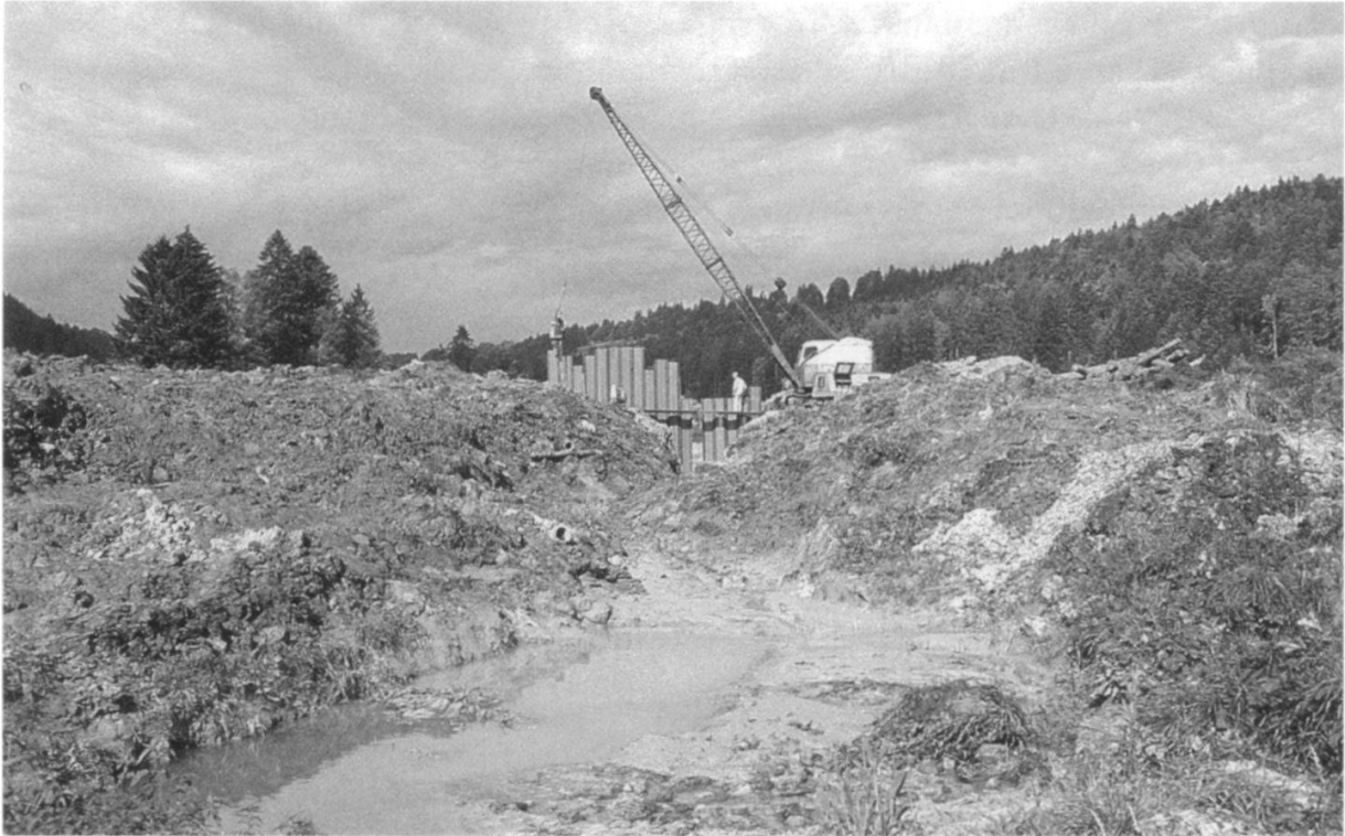
Figure 9: Pose des palplanches (Photo Fr. Gfeller, 7.9.1995).
