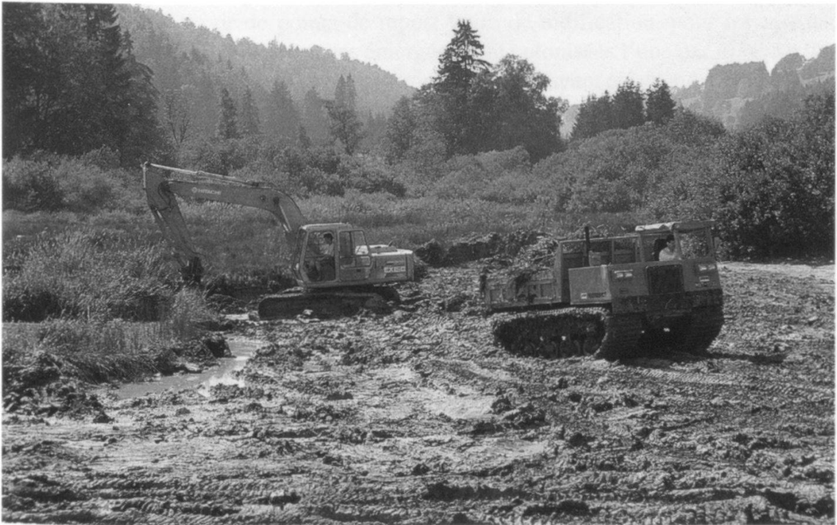
Figure 8: Travaux de creusage (Photo Fr. Gfeller, 10.8.1995).
