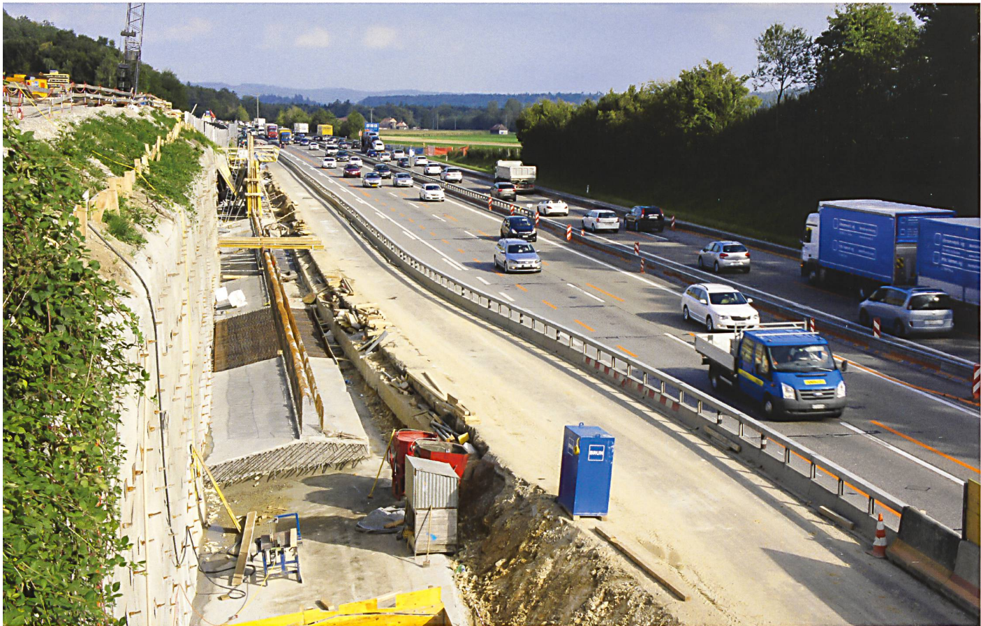
6-Streifenausbau der NA, Härkingen–Wiggertal, dem Born entlang
