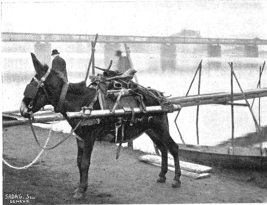
CHARGEMENT DE SUPPORTS.
