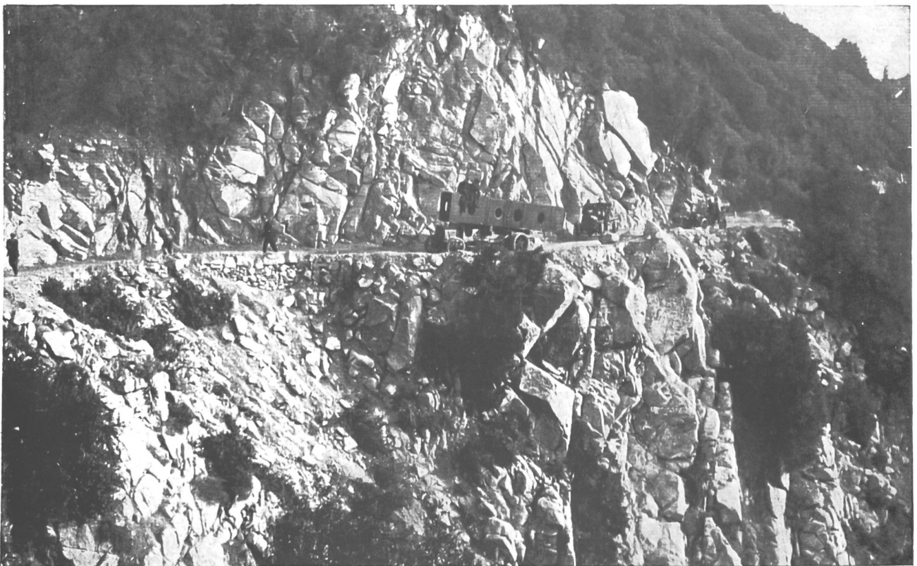
THE TRAIL AT MANY POINTS IS FRAUGHT WITH DANGERS THAT CALL FOR THE UTMOST COURAGE AND SKILL OF THE DRIVER. AT THIS POINT A LARGE BOULDER, WEIGHING 1,200 POUNDS, FELL FROM THE SIDE WALL, STRIKING THE GIRDER. NOTE THE BOULDER IN THE ROAD IN FRONT OF THE SECOND TRUCK
