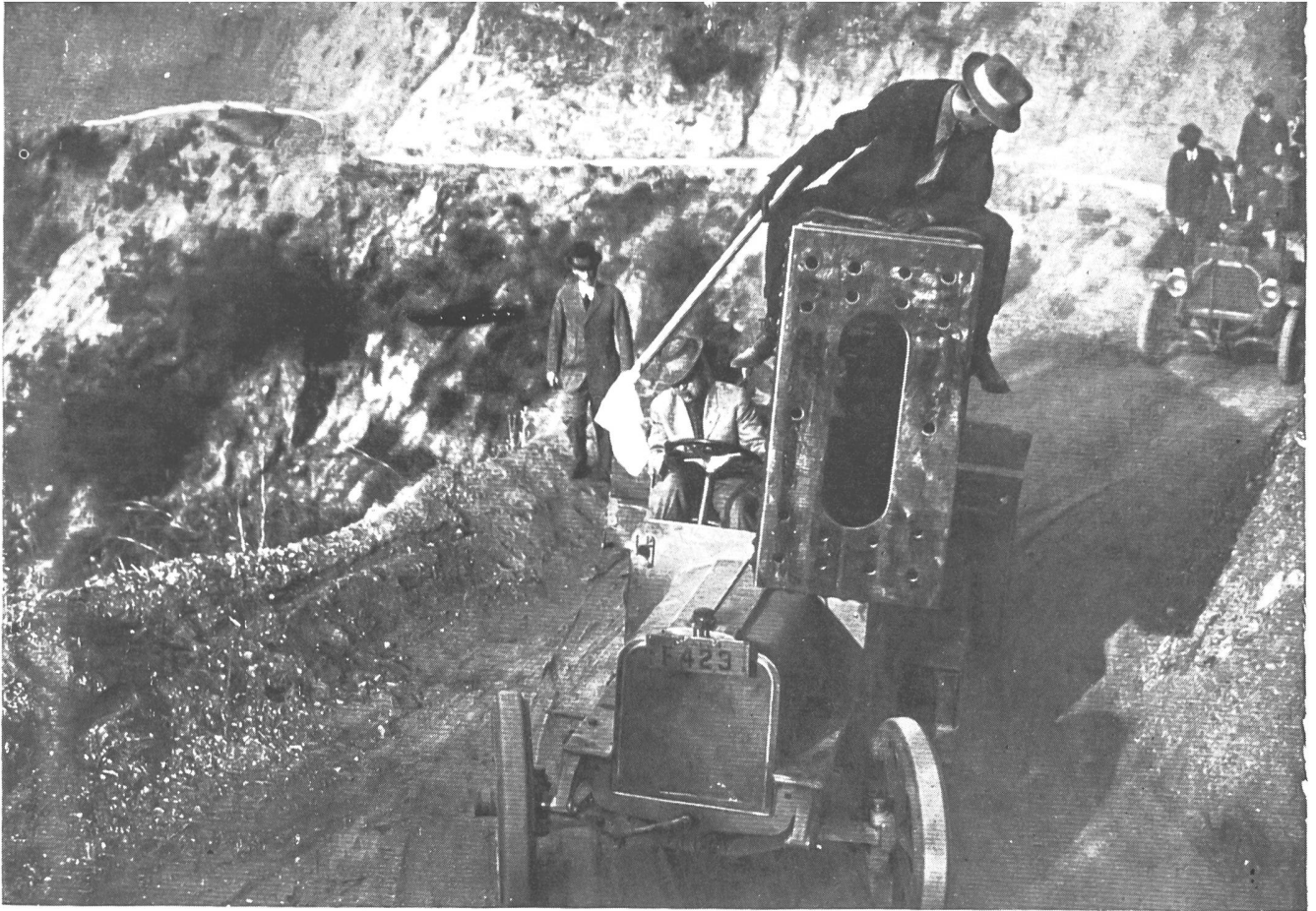
MAKING ONE OF THE SHARP TURNS, SHOWING ONE MAN PERCHED ON FRONT OF LOAD GUIDING MR. STONER WHILE DRIVING, AS THE 13-TON BEAM OBSCURES HIS VISION ON THE LEFT SIDE
