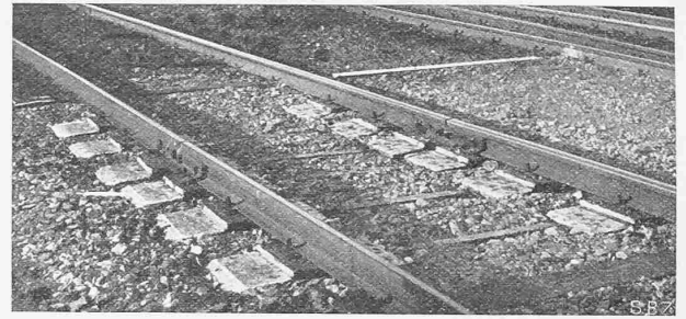
Abb. 1. Eisenbeton-Schwellen System Emperger.
