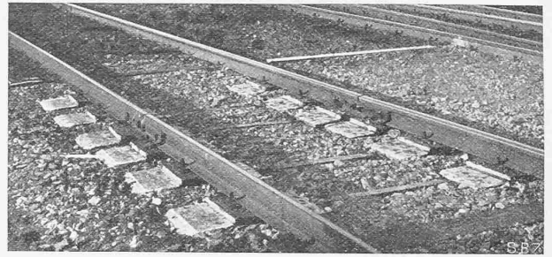
Abb. 1. Eisenbeton-Schwellen System Emperger.
