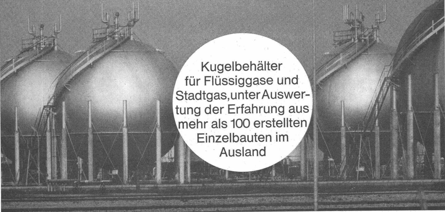
A black and white photograph of several large, spherical gas storage tanks. Each tank is supported by a complex metal structure of vertical columns and diagonal bracing. The tanks are arranged in a row, and the background is a clear, light sky. A tall, thin lamppost stands in the foreground between the tanks.
