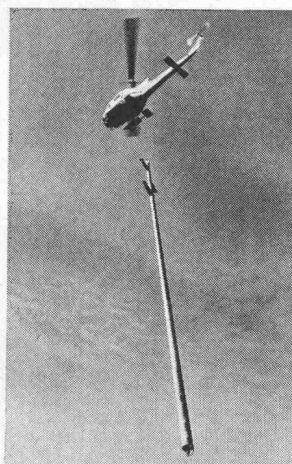
Transport eines 26-m-Mastes
