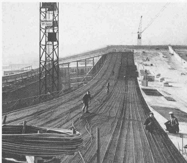
Bild 14. Armierung und prestressing steel for a 10 m wide strip of the suspended shell Reinforcement and prestressing steel for a 10 m wide strip of the suspended shell
