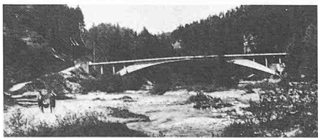
2051 Schwarzenburg 1932 Rossgrabenbrücke, Ing. Maillart Robert
