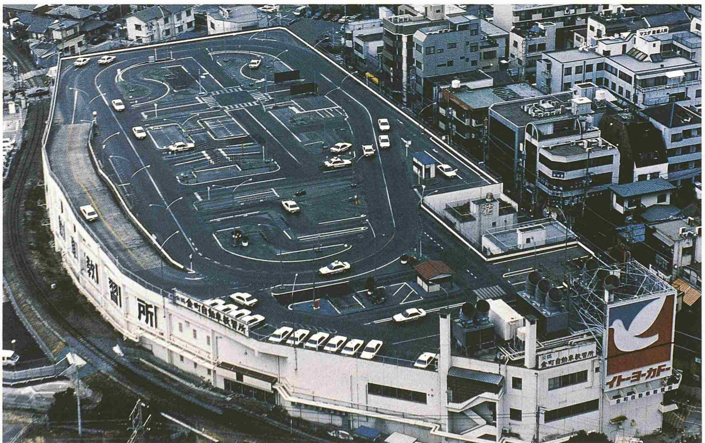
«Super car school»; function: supermarket + driving school/site: kanamachi, katsushika-ku: on top of the double layer supermarket lands a layer of driving school – the site includes the parcels of other people's property which could not be purchased – the condition of the site, framed by the curve of the railroad, is expressed directly in the extruded volume of the building – the entry ramp is framed above by the practice slopes for hand brake starts learner cars, etc.
