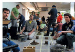
CArPE training site: clay and straw construction techniques CArPE Collectif d'architecture participative et écologique Lausanne
