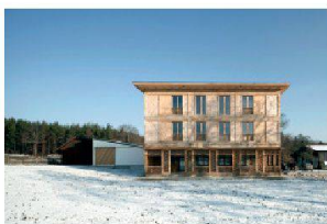
Building with pith-free hardwood bernath + widmer Architekten Zurich
