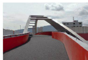
Railway overpass Zurich West huggenbergerfries Architekten Zurich
