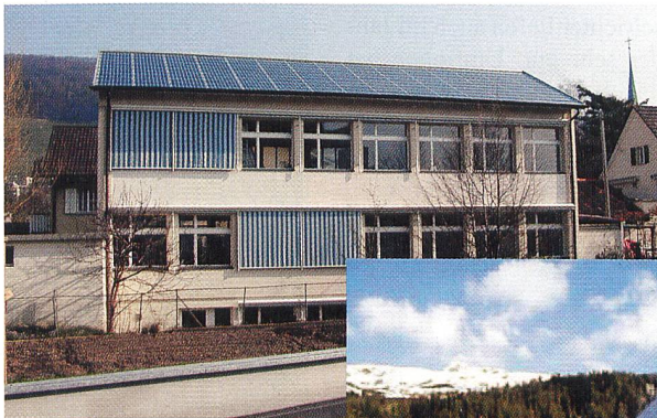
PV-Dachanlage in Wettingen (Photo NET AG).
